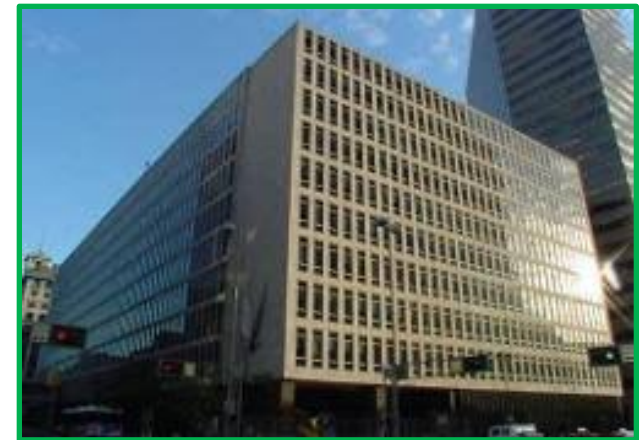
JW Peck Federal Bldg., Cincinnati, OH
